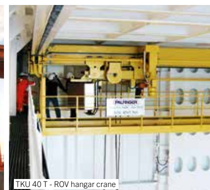
TKU 40 T - ROV hangar crane
