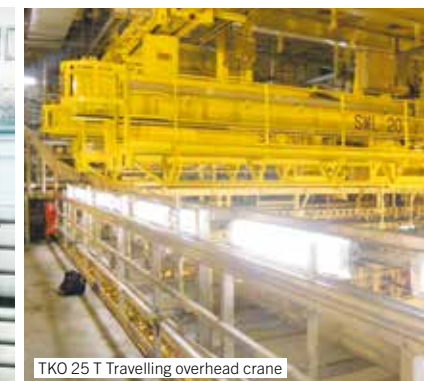
TKO 25 T Travelling overhead crane
